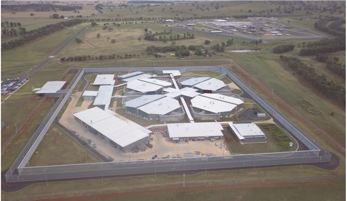
Macquarie Correctional Centre, Wellington, New South Wales
